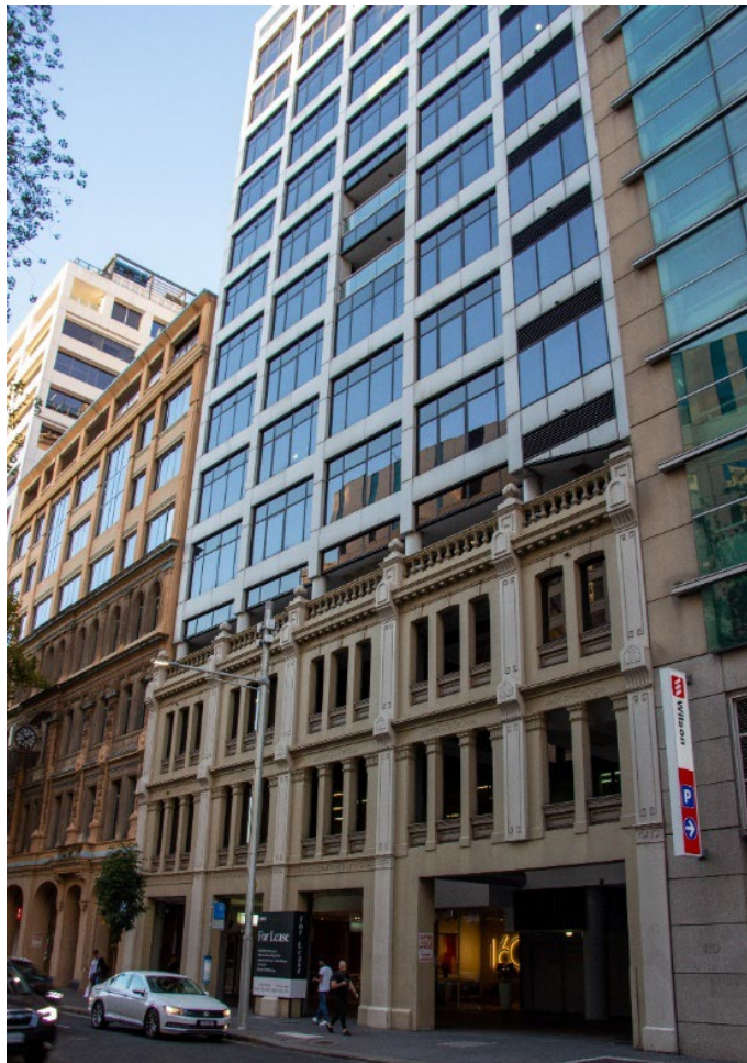
Figure 18 View along Sussex Street to the north
